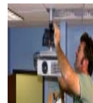
Pole Mount Platform Installation
